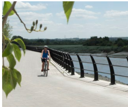
The riverside walk and bridleway at Peters Village
